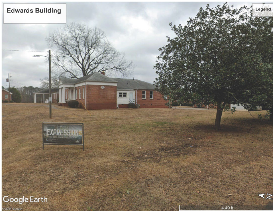
2. View of the Edwards building.
