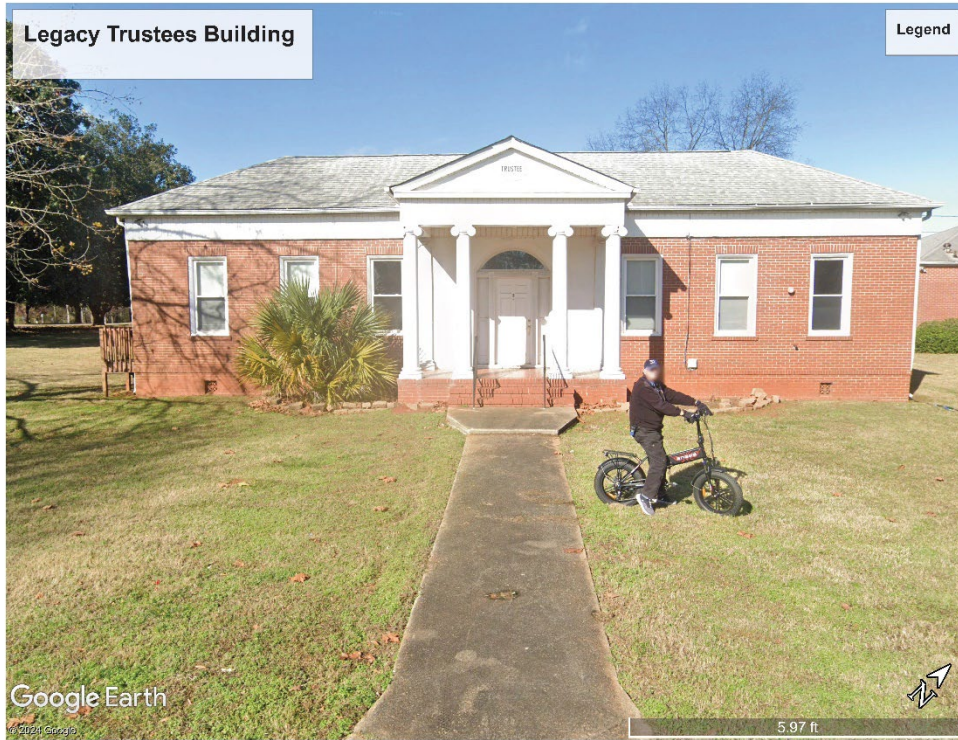
1. View of the Trustees Building.
